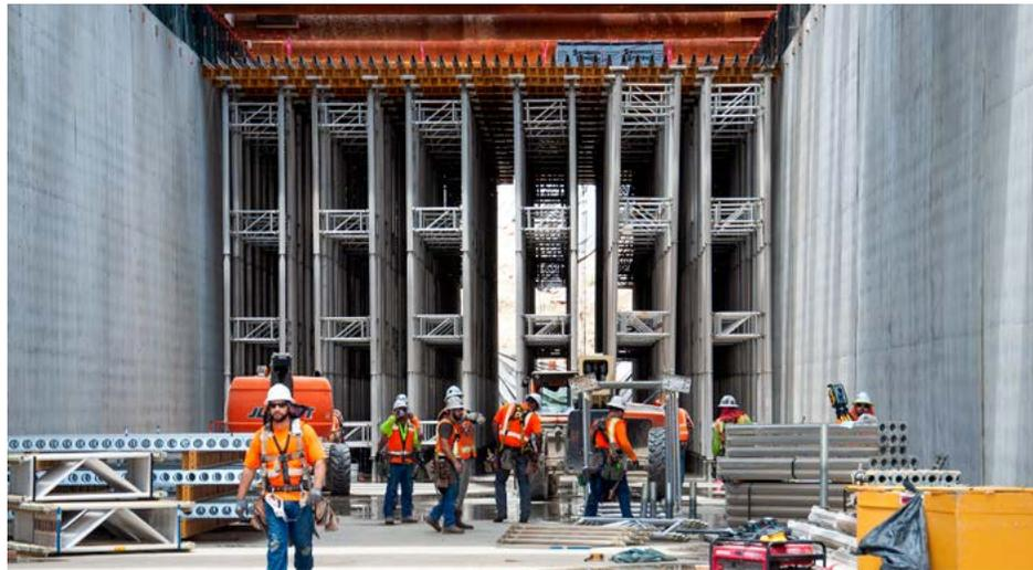
*California High-Speed Rail crews assembling scaffolding for the construction of a trench box lid.*
